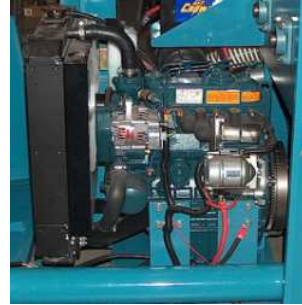
24.8 gross hp Kubota Diesel Engine
