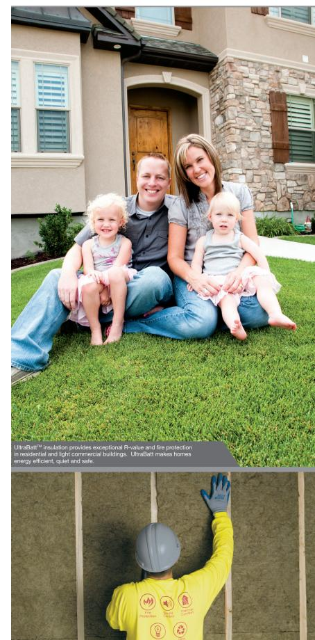
UltraBatt™ insulation being installed in a residential wood stud application. The semi-rigid batts are denser than traditional batts, making them easy to install.
