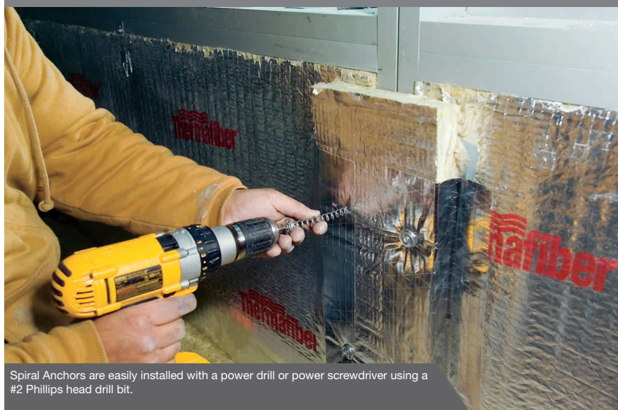
Spiral Anchors in conjunction with Impasse® hangers were used in the perimeter fire containment system in the Vdara hotel in Las Vegas.
