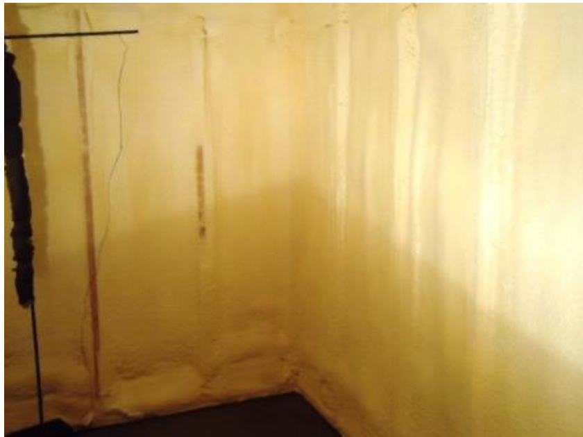
Opposite Corner Prior to Testing
