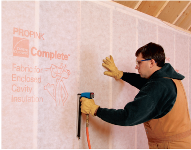
Fabric staples to studs quickly.
