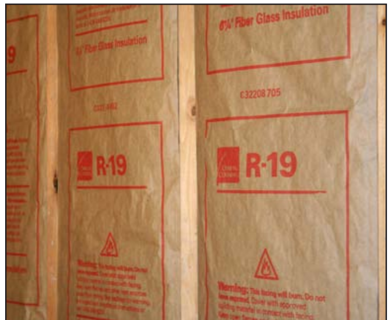
Properly installed inset-stapled fiberglass insulation, resulting in a Grade I rating.
