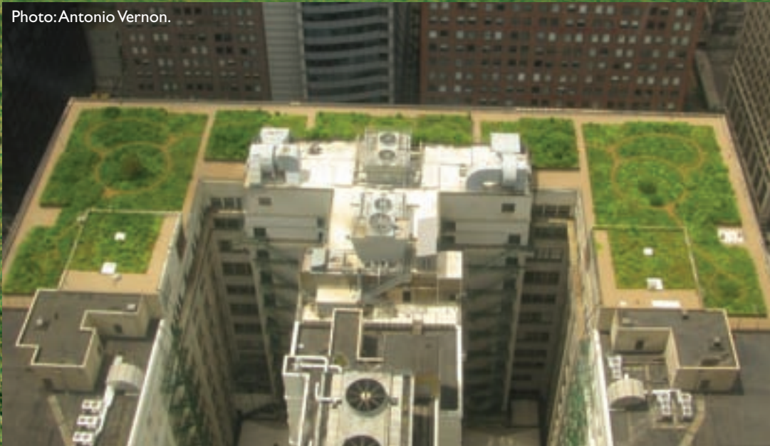
City of Chicago City Hall Green Roof Garden project.
