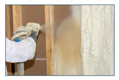
Open-cell Spray Foam (ocSPF) insulation is a great economic choice in insulation; it is a low-density (0.5lbs/ft) nonstructural insulation that offers excellent thermal and acoustical performance and high yields per drum set. When properly installed it expands 120 times its initial volume, sealing all voids, gaps and crevices, which makes it perfect for filling wall cavities of any shape and/or size.
