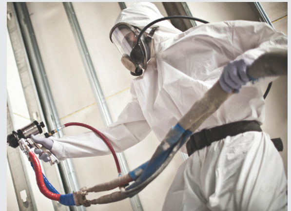
Install of JM Corbond oc SPF in commercial
