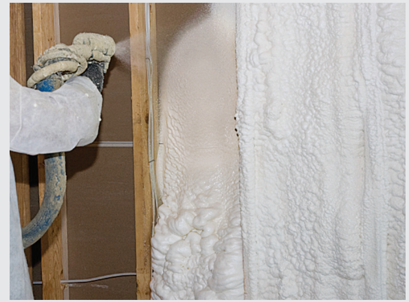
Install of JM Corbond oc SPF in residential
