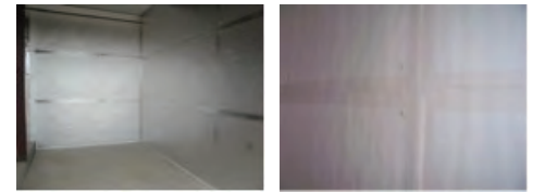
Interior Air Sealing with Tape
