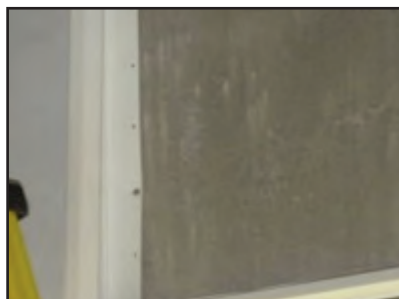
PVC attached to tilt-up wall
