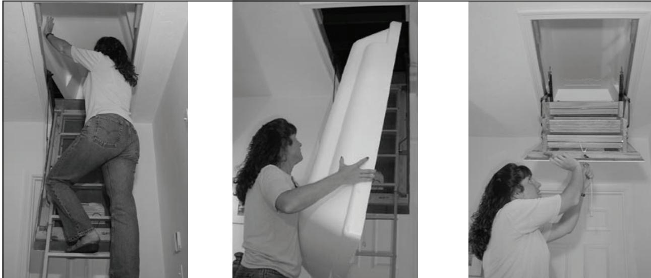
Draft Cap is lightweight, and easily installed in minutes. Made of durable dust-free expanded polystyrene foam, Draft Cap covers the attic stair opening to prevent air flow, and meets all local and federal energy codes for insulation.
